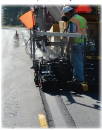
Built from heavy duty components and state-of-the-art electric heating elements, the Carlson Bolt-on Tapered Notch is able to give operators a longer attachment lifecycle while ensuring consistent performance and mat quality. The attachment is spring loaded so to no interfere with the screed's ride characteristics. And with the Tapered Notch's design, the attachment increases the material containment of the
